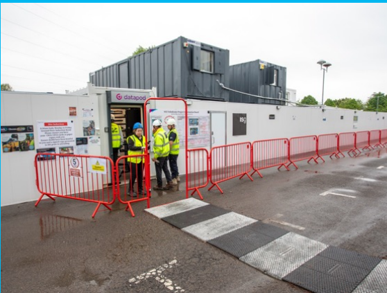
Crossing point with access gates
