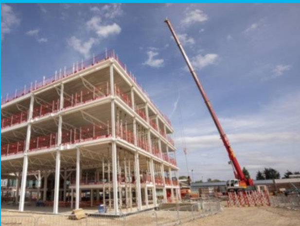
Mobile crane operations with robust exclusion zones
