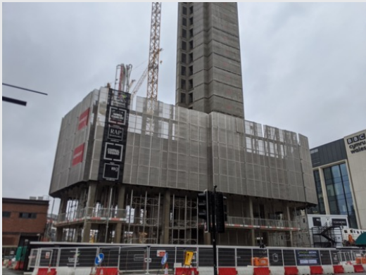
Safe screen utilised to eliminate falling objects
