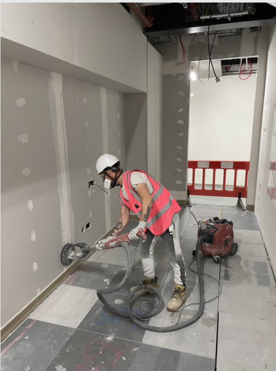
'M' class dust extraction in use
