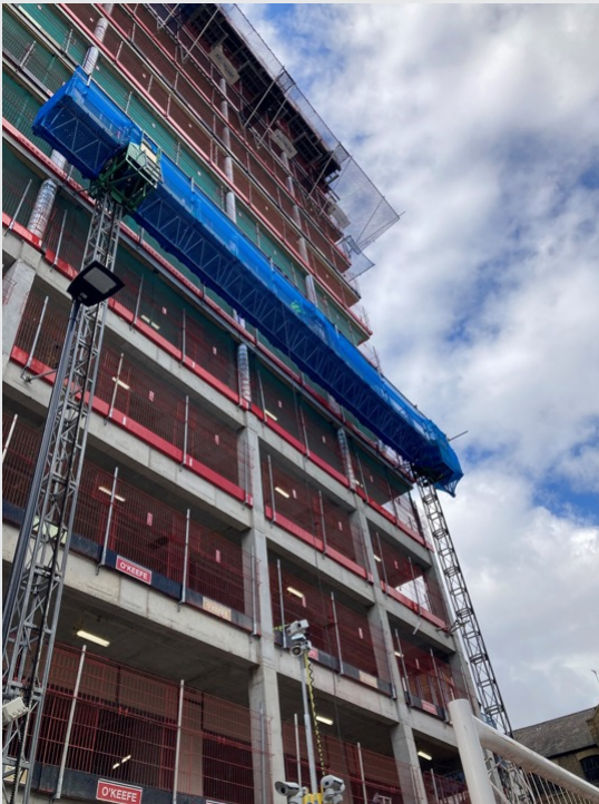
Mast climber with robust safety netting
