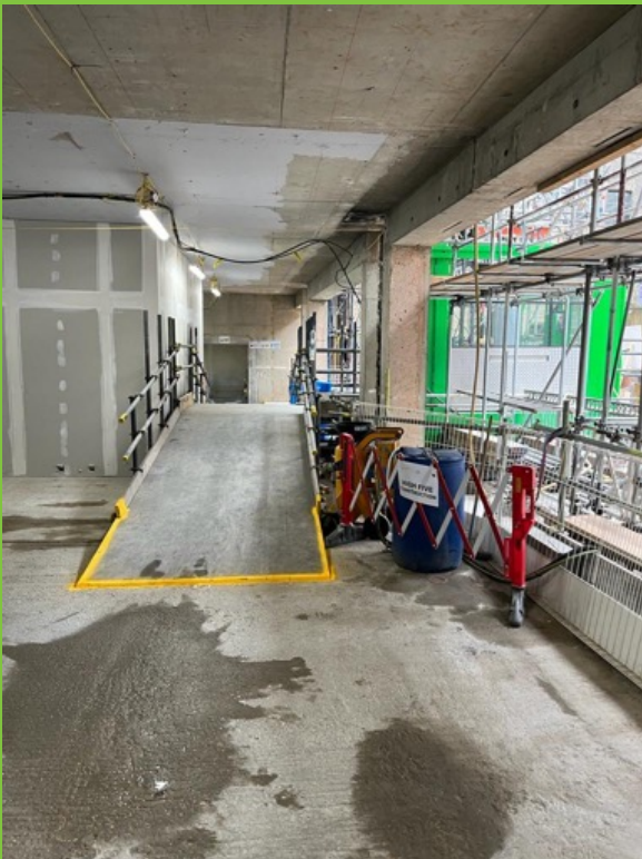
Fully designed access ramps
