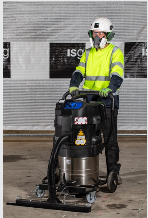
Clean-up operations with vacuum cleaner
