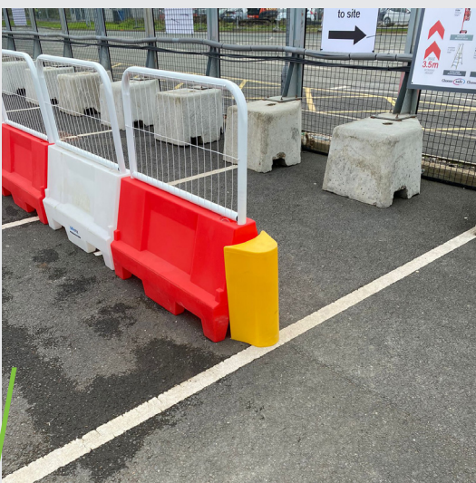
End protection installed where barriers present trip hazard (RB2000 shown)
