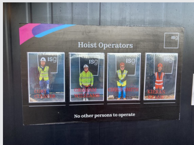
Example of signage to clearly display authorised hoist operators
