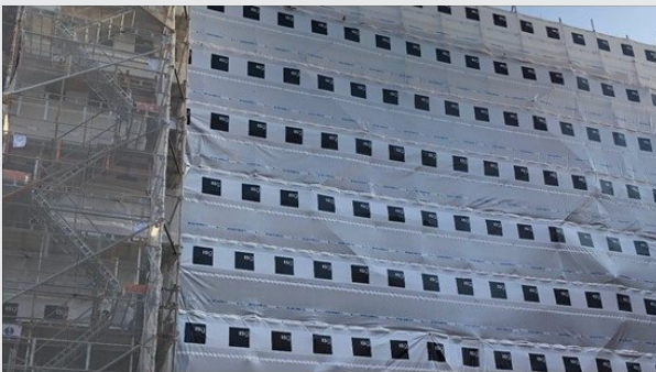
External scaffolding with full-height monoflex / containment netting
