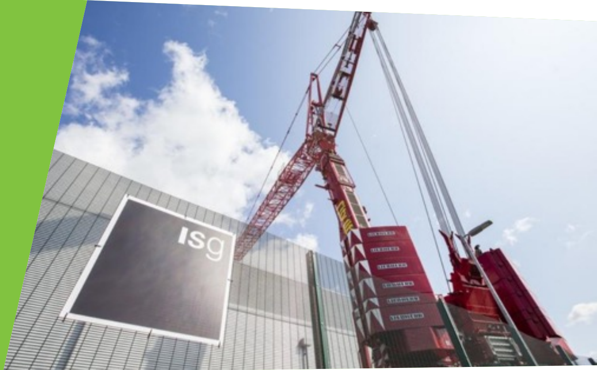
Mobile crane operations
