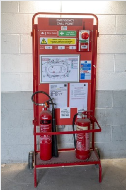
Good-practice examples of temporary fire points
