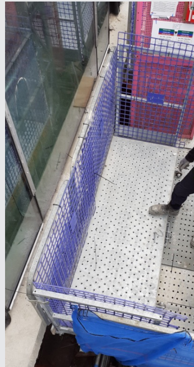
Roller decks designed to close gaps to façade
