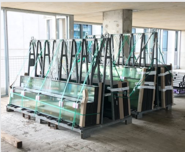
Glazing secured to stillage with individual banding
