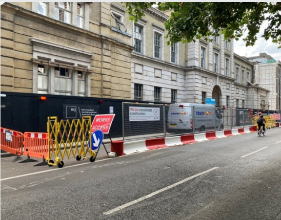
Segregated vehicle pit lane
