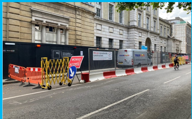
Pit lane providing segregation
