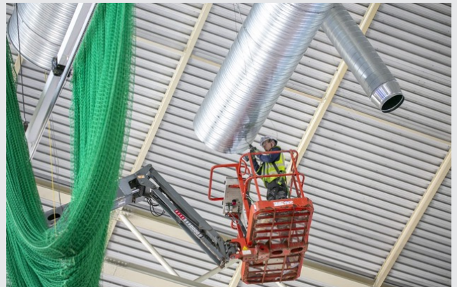
Boom lifter with operator wearing harness and restraint
