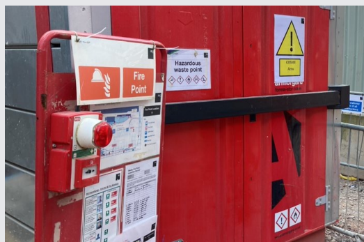
Example of a secure fully bunded COSHH store
