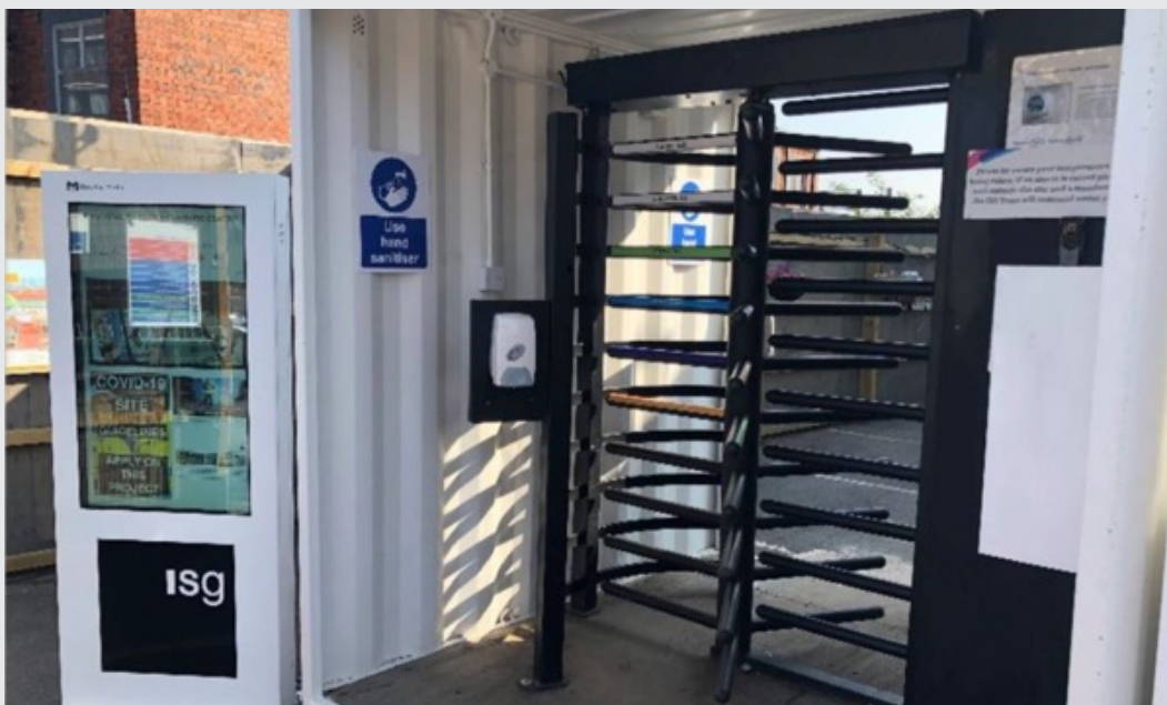
Turnstile complete with access control and information board
