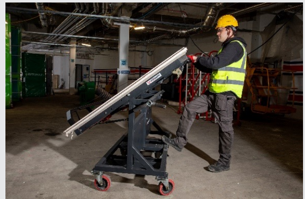
Rotating board trolley to provide safe storage and working bench
