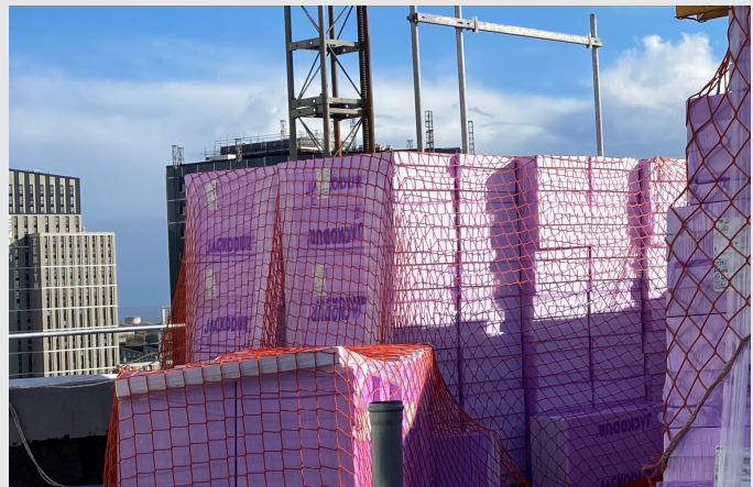
Lightweight materials secured at roof level with containment netting
