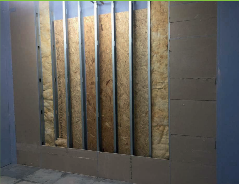
Plasterboard waste has been minimised by reusing off-cuts for first-fix patressing on internal walls and ceiling bulkheads
